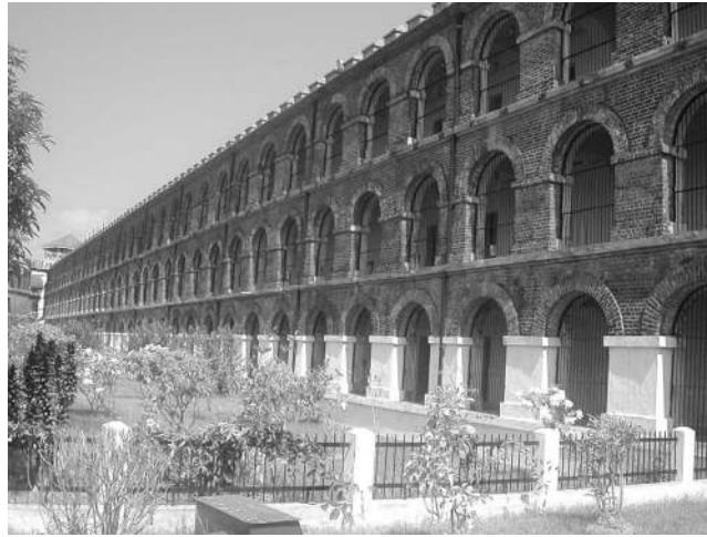
Figure 9. Undamaged three-story masonry structure of the cellular jail (photo: S. Jain).
