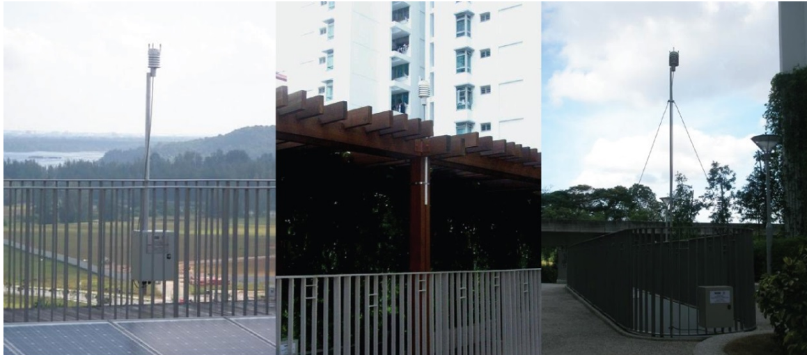
1 2 Figure 7: Installation of the weather stations (left: on roof; middle: on eco-deck trellis; right: on eco- 3 deck railing) (modified from Pan ShanShan 2 ).
