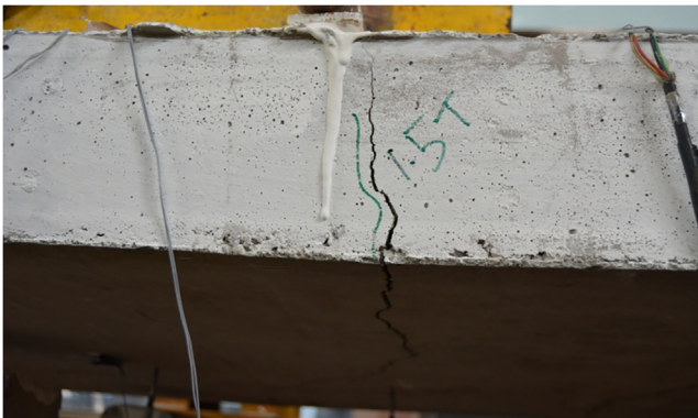
Fig. 6 Picture of failed panel F1.
