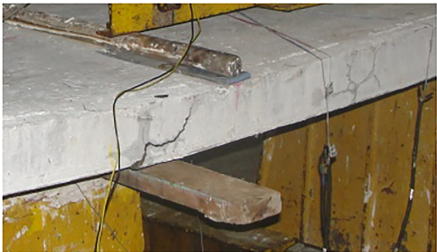
Fig. 7 Picture of failed panel F4.
