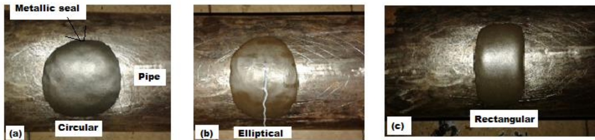
Figure 6. First phase repaired specimens of circumferential slot defect with different configurations (a) Circular (b) Elliptical (c) Rectangle
