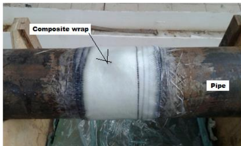
Figure 5. Circular defect repaired with elliptical configuration of metallic seal further reinforced with composite sleeve
