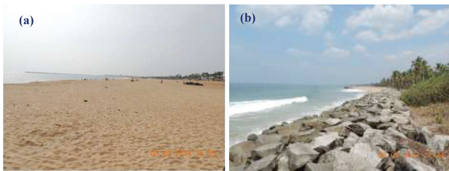
Fig. 3 (a) Wide beach to the south of Thangassery harbour and (b) Erosion along the Eravipuram-Thanni coastal sector located a few km to the south of the Thangassery harbour
