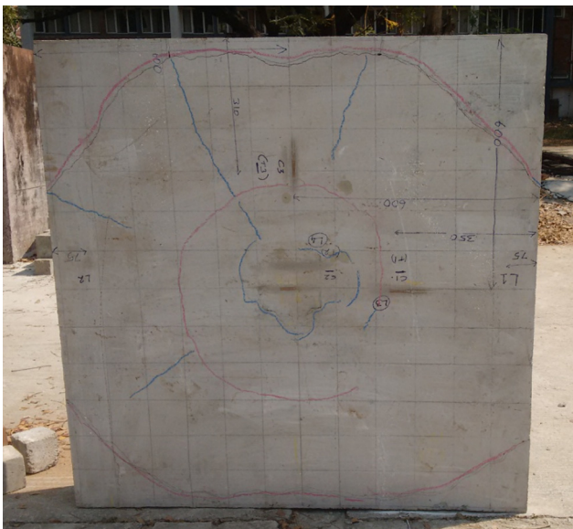
Figure 9c Cracks seen in top wythe (under punching load).
