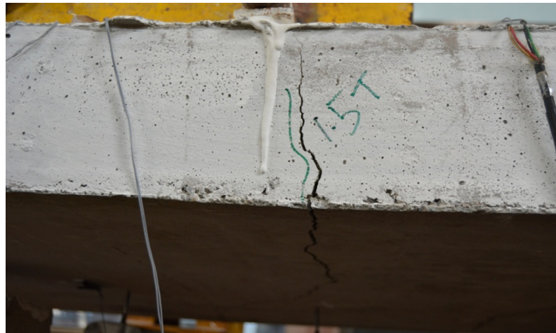
Figure 13 Crack seen in side and bottom of the panel (four-point bending test).
